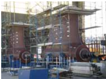
The propulsion pods under construction
