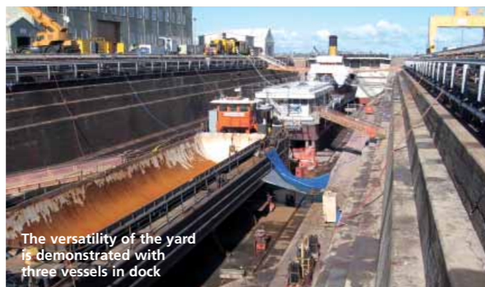
Main engines removed
