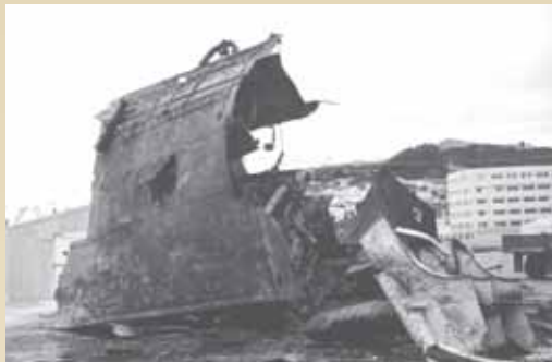
ABOVE: The stern engineroom section (with explosion hole) in August 1972. The final section was lifted ashore on March 29, 1973
